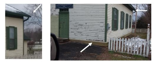
Shown are photos of the township's renovation of the Old Town Hall. Left photo shows the addition of the green gutters and downspouts. This is a first for the building. Right photo shows the foundation repair. Exterior painting will be done when (continued next page)
